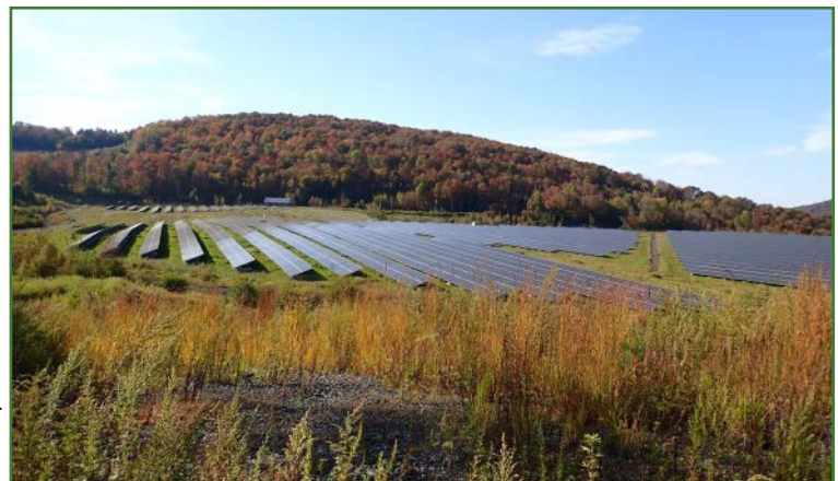
Solar array and restricted area as seen from Parcel 2.
