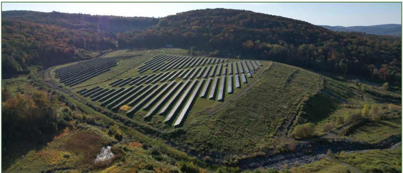
Solar array with view of the restricted area. Bottom right side is Parcel 2. Seen in background is old mine off property.
