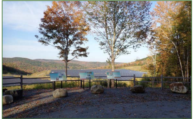
State info area showing solar array and view of Parcel 2.
